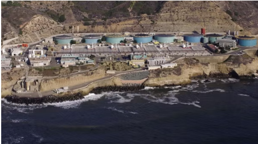
Sea level rise threatens many wastewater treatment facilities, such as this one in Point Loma (City of San Diego).
