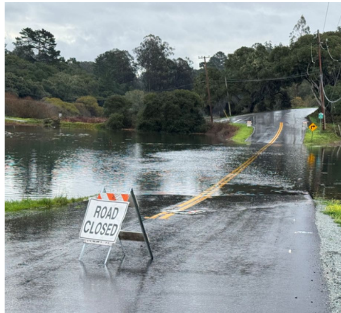
Storm and tidal flooding threatens many coastal roads, such as this one in Monterey County (CA King Tides Project).
